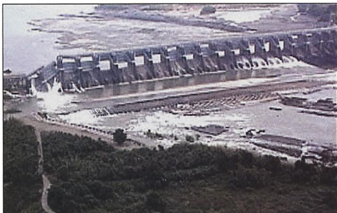
Fault surface rupture across Shigan Dam.
