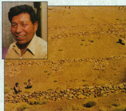
Stone walls trap water (Inset: Norphel).
