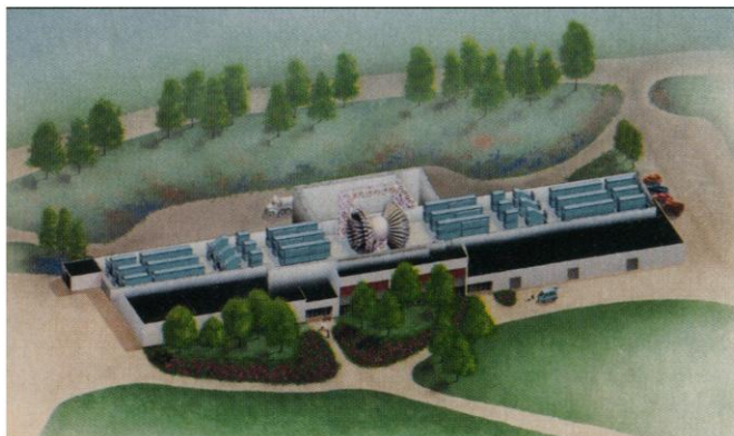
The big squeeze. An artist's conception of the National Ignition Facility, which would focus 190 or more laser beams on tiny pellets of hydrogen to fuse them into helium.
