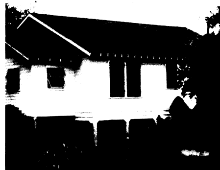
"Subsidence of an organic soil (in this case a Saprist) has lowered the ground surface around the pilings and around the septic tank of this house at the Everglades Research and Education Center, Belle Glade (Gold Coast-Florida Bay physiographic district). The ground surface originally was just below the floor of the house." [From Brown et al. 's chapter in Ecosystems of Florida ; photo by R. B. Brown]
