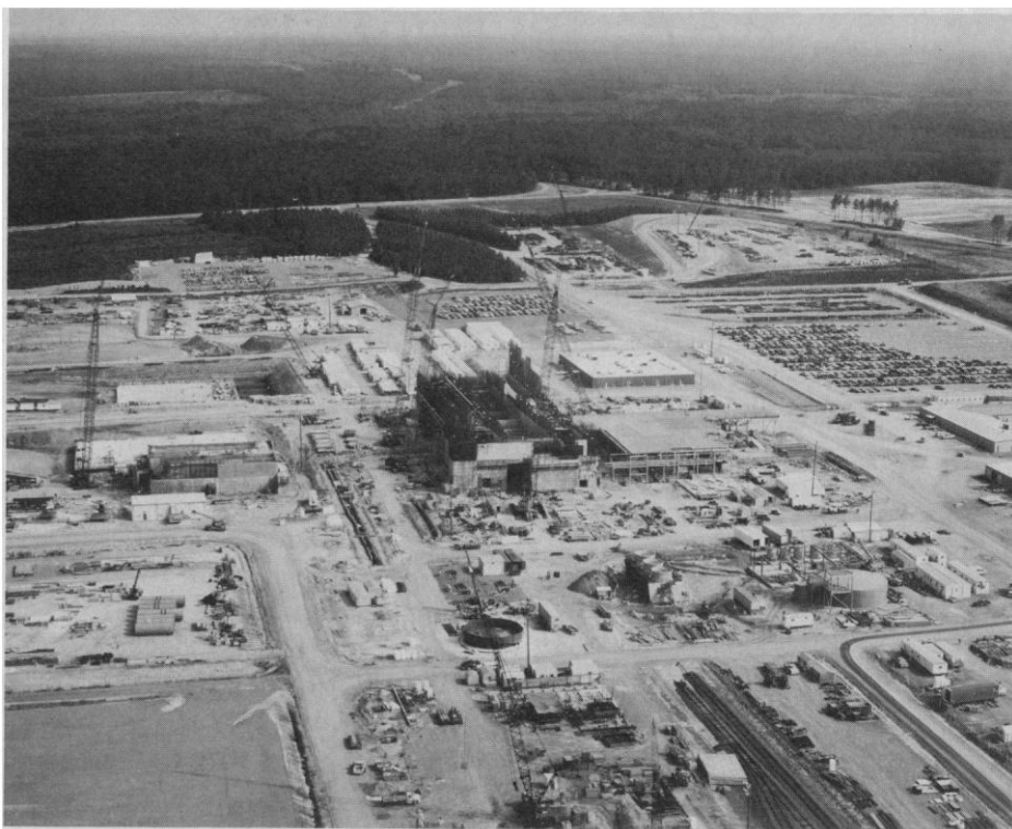
Savannah River's newest addition. At the center is the heart of the Defense Waste Processing Facility, the glassification plant. Behind, at left, are the foundations of the storage building that will hold 2300 canisters (5 years' output) of "hot" glass.
