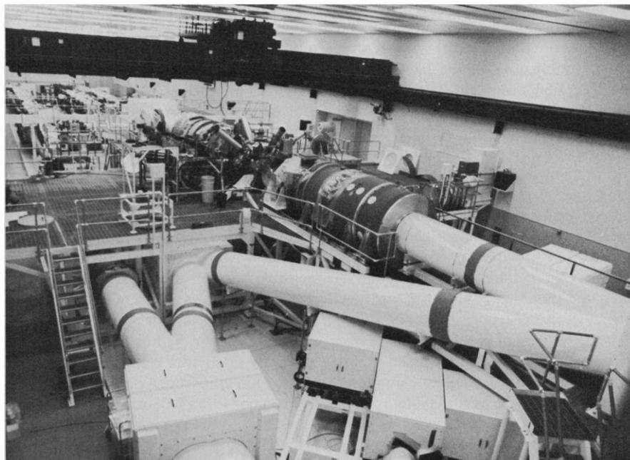
Fig. 2. The Novette laser, a harmonically converted Nd:glass laser that generated 9 kJ of 0.53- $\mu\text{m}$  light and 1.5 kJ of 0.26- $\mu\text{m}$  light for short-wavelength laser-plasma experiments. In August 1984, its two beams were removed and installed as two of the ten beams in the Nova laser, which was completed in December 1984 and is now being activated.
