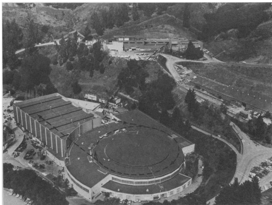
Fig. 1. The Bevalac complex. The dashed line indicates the path of a heavy ion from the SuperHILAC (top of photograph) to the Bevatron, where final acceleration occurs.
