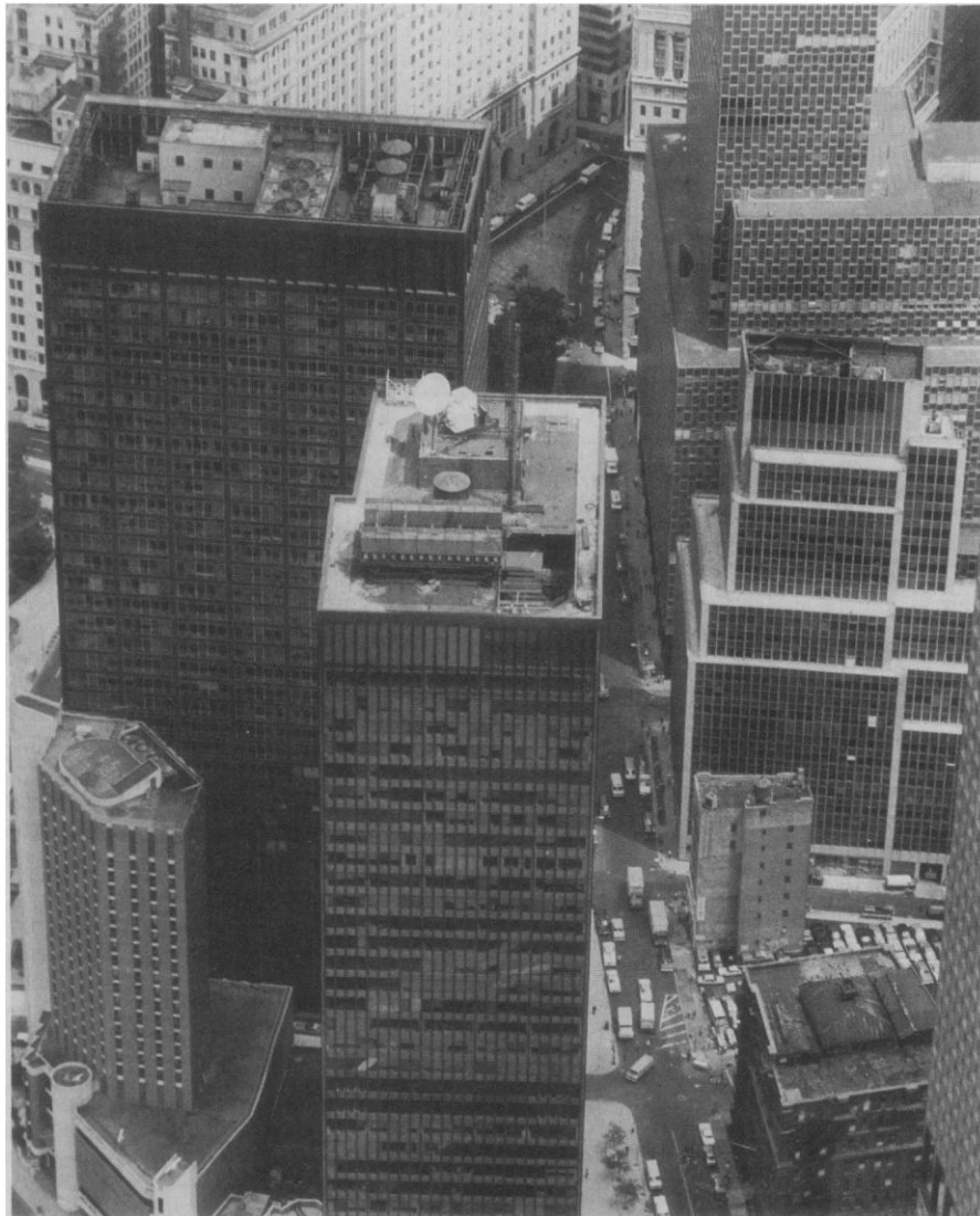
Fig. 2. Satellite Business Systems earth station with aperture 5 meters, transmitted power 500 watts, and throughput 12 Mbit/sec. This station is located on the roof of One State Street, New York City.
