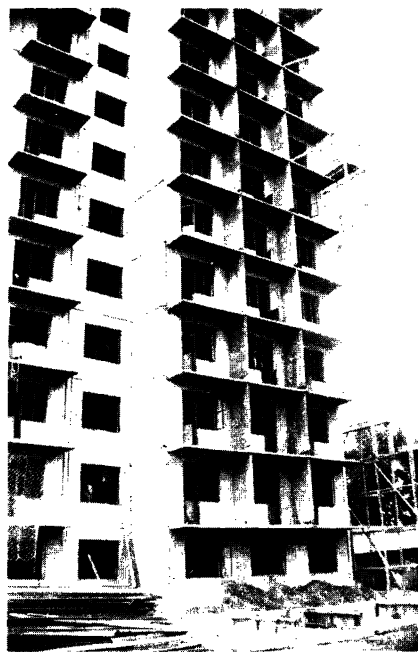
A 12-story apartment building under construction in Beijing (Peking). "Buildings in Peking are designed by the Peking Institute of Architectural Design for an earthquake of intensity VIII on the Chinese scale." This and a similar project visited "seemed to typify new apartment construction in Peking." It "has precast exterior walls, precast floors with topping, cast-in-place concrete shear walls, and brick partitions." With the construction procedures used, "it takes approximately 2 months to finish the concrete construction and about six months for total building completion." [From Earthquake Engineering and Hazards Reduction in China ]
