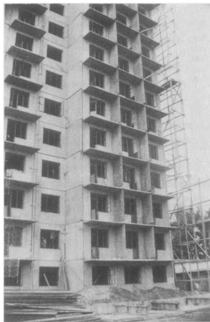
A 12-story apartment building under construction in Beijing (Peking). "Buildings in Peking are designed by the Peking Institute of Architectural Design for an earthquake of intensity VIII on the Chinese scale." This and a similar project visited "seemed to typify new apartment construction in Peking." It "has precast exterior walls, precast floors with topping, cast-in-place concrete shear walls, and brick partitions." With the construction procedures used, "it takes approximately 2 months to finish the concrete construction and about six months for total building completion." [From Earthquake Engineering and Hazards Reduction in China ]
