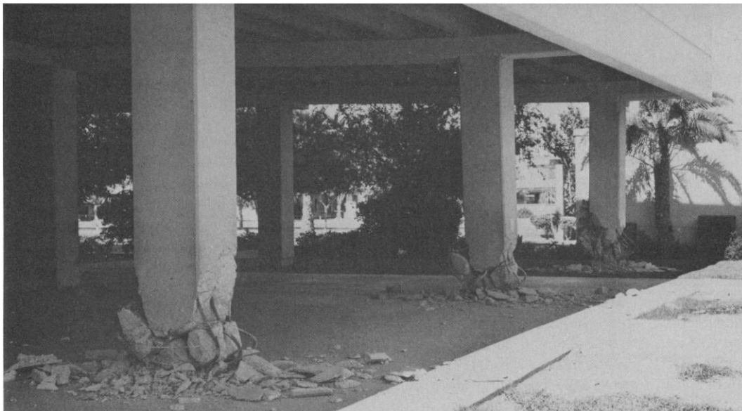
Columns at the eastern end of the Imperial County Services Building after the Imperial Valley earthquake of 15 October 1979. The rocking and swaying of the five upper floors shortened the eastern columns, but no others, by about 20 centimeters. The wall in the left of the picture and three similar walls helped resist the shaking, but they were too far from this end of the building to save these columns. The building will be demolished, according to county officials. [Photo by John Robb]
