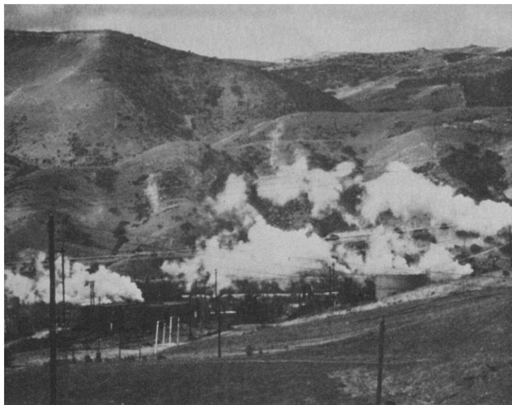
Injection of steam is already being used to increase production of heavy oil, as in the San Ardo field in California. [Source: Department of Energy]
