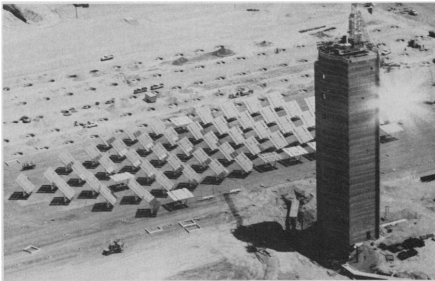
Fig. 1. The $21 million power tower test facility at Albuquerque, New Mexico. Seventy-eight sun tracking mirrors or heliostats are in place, and eventually 200 more will be added. The mirrors focus sunlight on the top of the 200 foot tower, on which experimental boilers will be tested. Note the pickup trucks in the background to indicate the scale of the facility.
