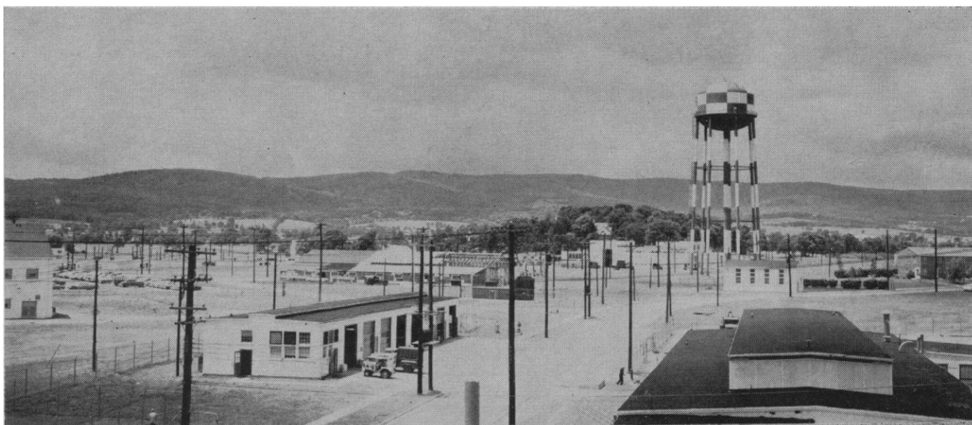
A portion of Fort Detrick looking west into the Catoctin Mountains.
