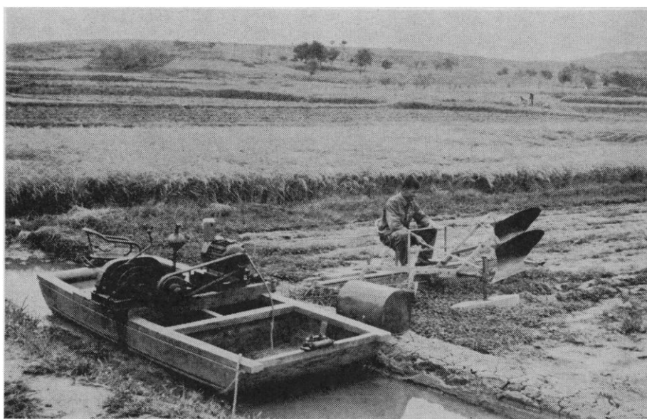
Fig. 8. The cable-towed plough designed at the Agricultural Mechanization Research Institute, Nanking. Here the winch on the boat is powered by an electric motor.
