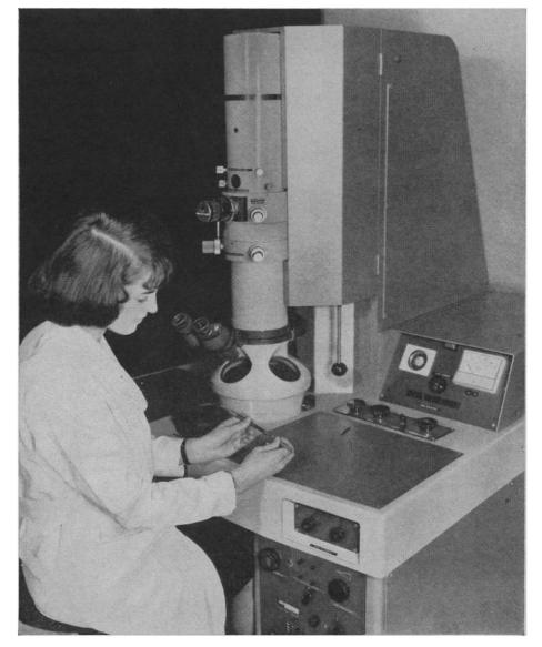
**FULLY AUTOMATIC PHOTOGRAPHY:** At the touch of a single lever the automatic sheet film camera produces properly exposed, sequentially numbered 2¾ x 2¾ inch micrographs. Film transport is automatic, thus double exposure is impossible.
