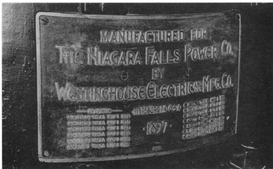
Fig. 5. A recent photograph of the nameplate of one of the earliest generators at the first great Niagara Falls plant. Nine of Tesla's patents are listed. [Courtesy of the Niagara Mohawk Power Corp.]
