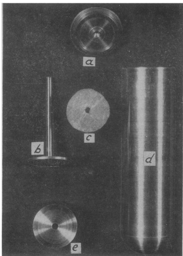
FIG. 2. Centrifugal tissue mincer disassembled.
