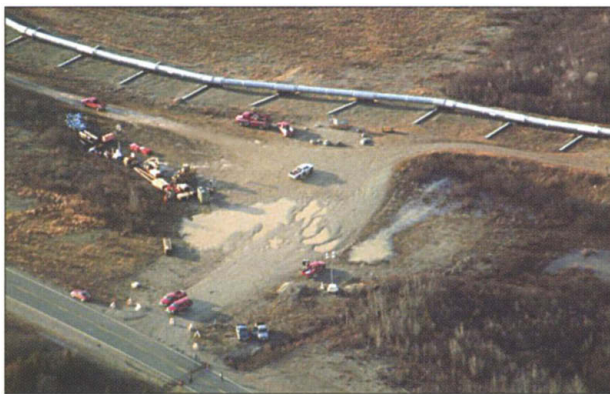
Not a drop. The quake on the Denali fault, which broke through the highway at lower left, could not rupture the trans-Alaska oil pipeline.
