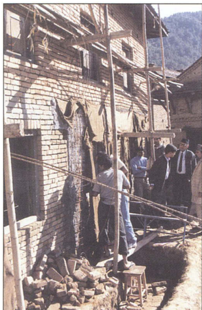
Pitching in. Working with donated labor and supplies, GHI helped a community strengthen this school in Katmandu, Nepal.
