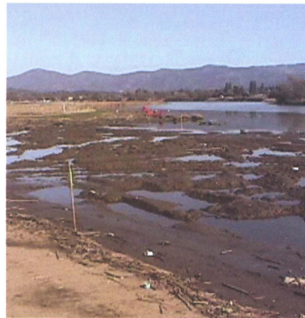
Investing in a living river. The residents of Napa, California, accepted higher taxes to pay for natural flood protection. Levees and dams along the Napa River were removed so that high waters will spill over onto the historical floodplain.
