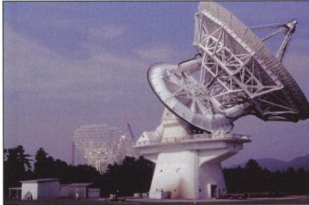
**Out with the old.** The National Radio Astronomy Observatory 140 Foot Radio Telescope during its last scientific observing run, July 1999. The Robert C. Byrd Green Bank Telescope is seen during construction in the background.
