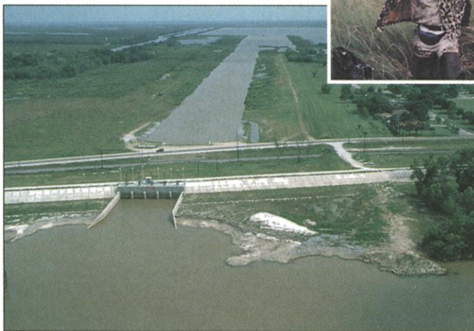
Necessary diversion. Planners hope to stem the loss of wetlands by spilling water from the Mississippi River back into the marshes. A prototype is the Caernarvon Freshwater Diversion, 16 km south of New Orleans; since it began operation, some of the marshes of Breton Sound have rebounded ( inset ).
