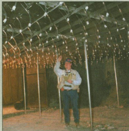
Slow drip. Water leaks faster than expected into the proposed Yucca Mountain repository.
