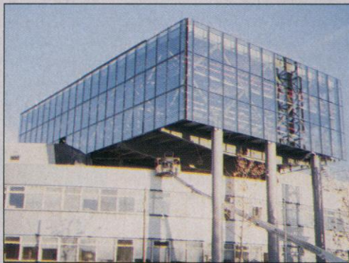
High security. Lyons's level-4 lab will sit over the old Pasteur Institute building.
