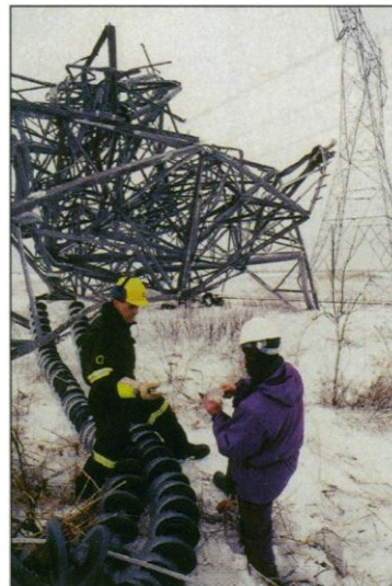
Nature 1, Quebec 0. Transmission tower was no match for ice storm.
