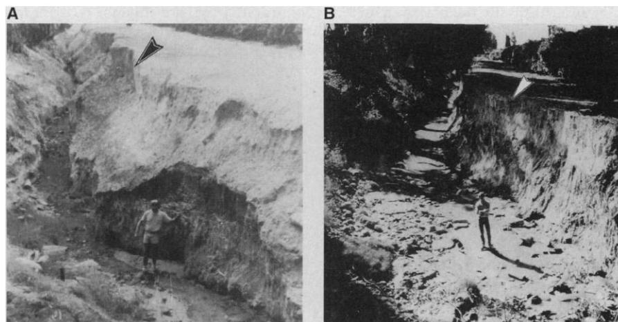
**Fig. 2.** An example of stream channel erosion in Hicks Canyon Wash, looking southeast at the confluence with Rattlesnake Canyon Wash (Fig. 1). (A) 1979. (B) 1993. A person stands at approximately the same location in both photographs. Note the retreat of the cut bank to the right. Arrows mark the location of surveyed profiles in 1983 and 1993 (Fig. 3).
