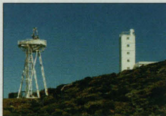
No vacuum here. Dutch "open" solar scope.
