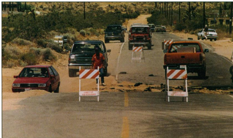
Shifting science. An earthquake that struck in 1992 caused this rupture, which shifted Reche Road in Landers, California. After the rupture, the edge of the far section was aligned with the center line of the near section. Knowledge of how such earthquakes are initiated may reveal whether the existence of a preparatory stage could be used for earthquake prediction. [AP/Wide World]
