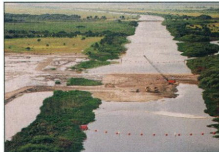
River test bed. Last year, as part of the Kissimmee River test restoration, high embankments were lowered ( left ). By last month, the area (shown at right from a different angle) had been transformed back into a flood plain, and patches of wetland vegetation began to recolonize it.
