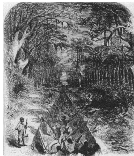
"Canal at Delta Point, 1862. Laboring in blistering heat, 1,200 slaves toiled alongside Union soldiers in an aborted attempt to bypass Confederate guns by cutting through a bend in the Mississippi River near Vicksburg." [From Structures in the Stream ; courtesy of the Boise Public Library]
