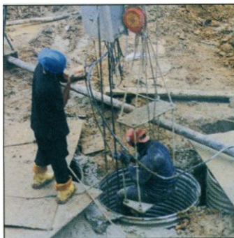
Getting into it. Laborer enters "tie-down" casing to prepare for drilling.
