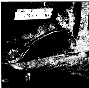
A nonfatal flaw. The Northridge quake cracked joints in steel-frame buildings, although none collapsed.
