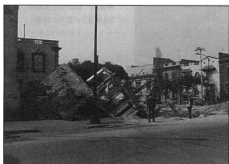
"Example of overturned building due to foundation failure in the 1985 Mexico earthquake. Here the piles were pulled out together with the intervening soil." [From Fundamentals of Earthquake Prediction ]
