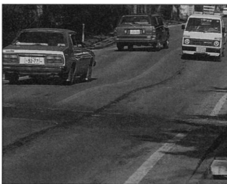
"A jinami or 'frozen' gravity wave photographed on soft ground after the 1987 Chiba, Japan earthquake." [From Fundamentals of Earthquake Prediction ; photo courtesy of H. Nirei]
