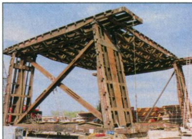
Why didn't someone think of this? Retired flatcars make 4-lane bridge; cross braces are old boxcar beams.
