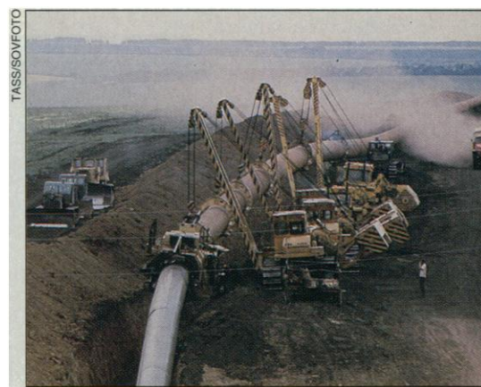
Leak prone. Laying a Siberian gas pipeline.
