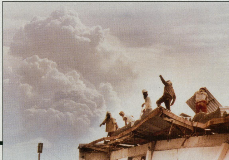
A dirty killer. Many died when rain-soaked ash collapsed roofs.
