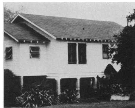
"Subsidence of an organic soil (in this case a Saprist) has lowered the ground surface around the pilings and around the septic tank of this house at the Everglades Research and Education Center, Belle Glade (Gold Coast-Florida Bay physiographic district). The ground surface originally was just below the floor of the house." [From Brown et al. 's chapter in Ecosystems of Florida ; photo by R. B. Brown]
