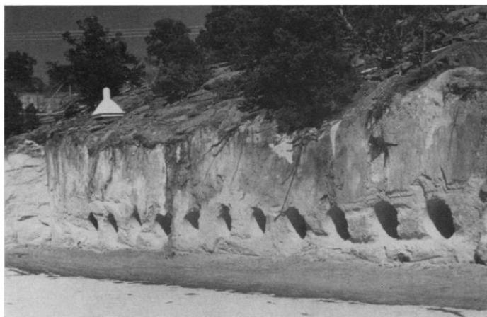
**Fig. 6.** Photograph of a portion of the "Cygnus" air shower array at Los Alamos showing drilling for underground muon detectors (courtesy of J. Goodman).
