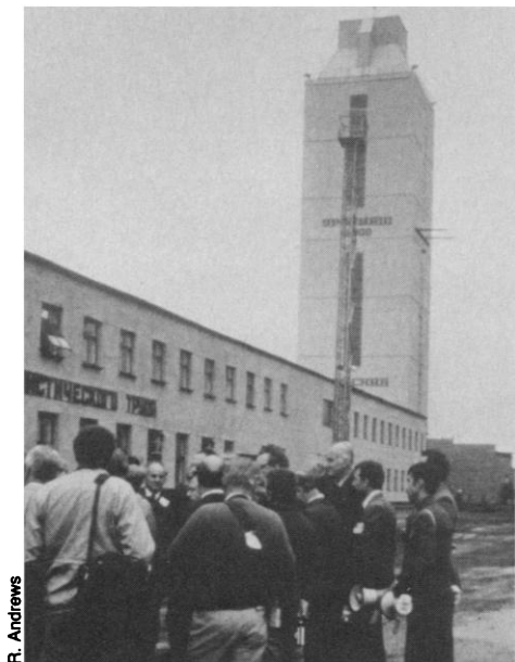
The Soviet ultradeep hole. This drill rig enclosure stands over the 12-kilometer-deep hole on the Kola Peninsula.
