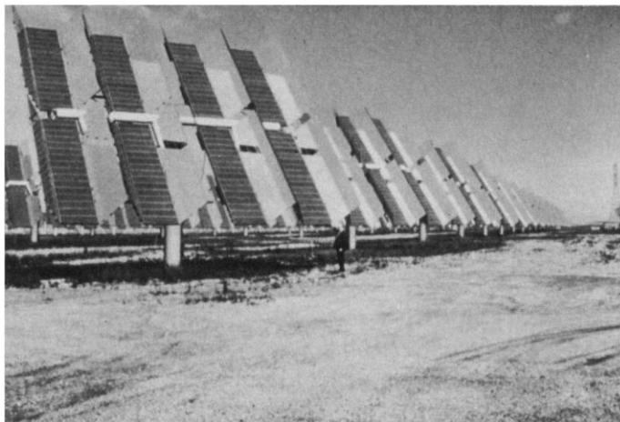
**Fig. 6.** ARCO Solar's 6.5-MW PV plant on Carissa Plains in California is the largest PV facility in the world. The arrays use mirrors to augment the sunlight impinging on the cells. [Courtesy of ARCO Solar, Inc.]
