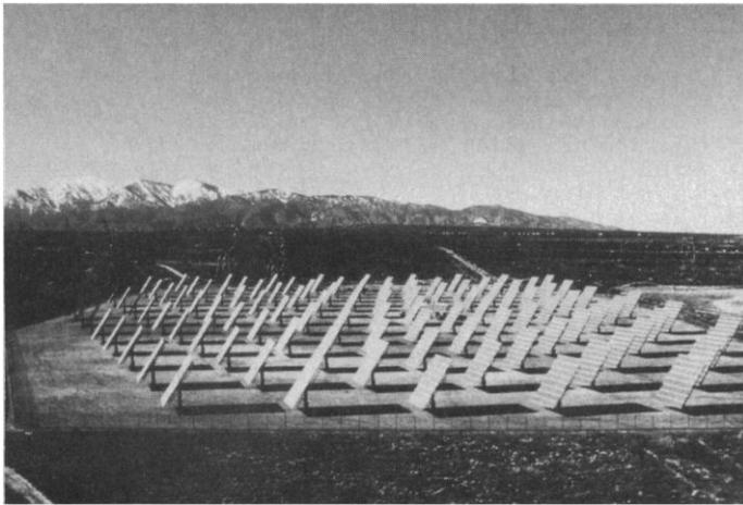
**Fig. 7.** The 1-MW PV plant on Hesperia Plains in California, built by ARCO Solar, Inc., in less than 1 year from inception. [Courtesy of ARCO Solar, Inc.]
