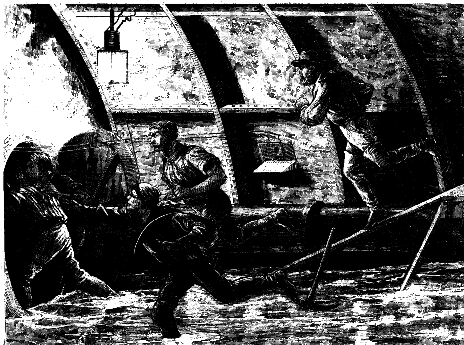
"Blow in Haskin's tunnel under the Hudson River (1880)." Blows (sudden loss of air pressure followed by inrush of water) occurred in a number of early compressed-air tunnels. In this instance, "the miners took refuge in the air lock, but one of the doors was jammed . . . and twenty men were drowned." This contemporary print shows the airlock on the left. Haskin's tunnel "is thought to be the first in which telephones were used . . . although the . . . wires must have been routed in a different way from that shown by the artist otherwise they would have been cut the first time the air lock door was closed!" [From Innovation and the Rise of the Tunnelling Industry ; Smithsonian Institution]
