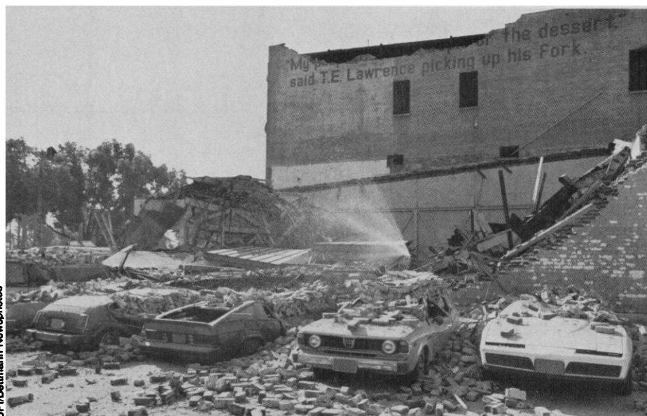
Brick can be bad. A single-story, turn-of-the-century brick building in Pasadena did not fare well during the Whittier earthquake. Such unreinforced masonry structures are prone to collapse during even moderate shaking.
