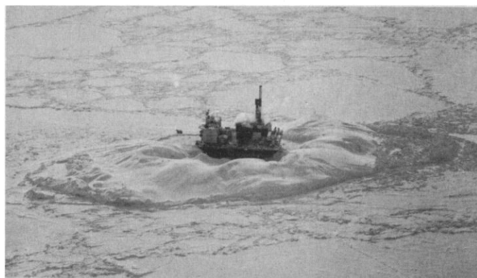
Fig. 2. Concrete Island Drilling System (CIDS) about 10 miles off Cape Halkett, Beaufort Sea coast, Alaska, 27 March 1985. The thick ice was a protective barrier created by pumps spraying seawater around CIDS except for an opening at the back of CIDS to egress. The deck of CIDS measures 295 × 312 feet (90 × 95 m) and is about 45 feet (14 m) above sea level; the ice barrier averaged about 60 feet (18 m) high and rested on the sea floor at a depth of about 50 feet (15 m). [Photo by Air Photo Tech, courtesy of Exxon Company, U.S.A.]
