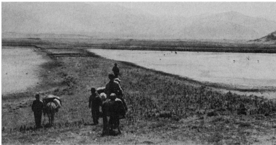
"A causeway, a raised earth roadbed, passes through a small lake by the Inka center Huánuco Pampa in the central Andes of Peru." [From The Inka Road System ]
