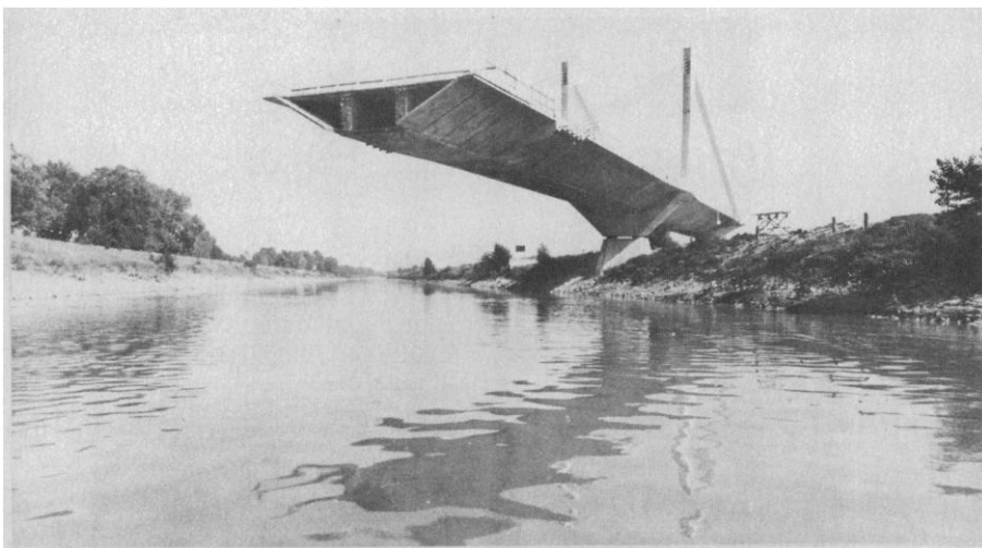
Strallato Bridge, near Vienna, a cable-stayed bridge under construction May 1979. Though the columns seem like cantilevers supported at the bottom, they are "actually elastically supported by the cables at the top. This elastic support not only restricts longitudinal movement of the column top, but also reduces the lateral buckling effect. This action has enabled designers to omit the expensive braces between the columns." [L'Industria Italiana del Cemento; from Lin and Redfield's paper in Long-Span Bridges ]
