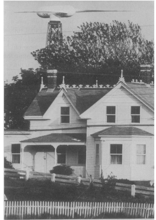
This DOE windmill on Block Island, Rhode Island, is one of four 200-kilowatt prototypes. Operating at wind speeds of 18 to 34 miles per hour, it produces about 10 percent of the island's power supply.
