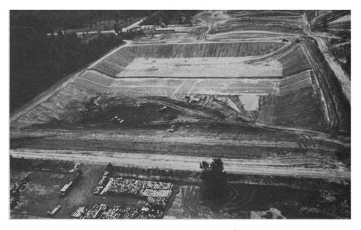
HDPE is fused onto the surface of the wastes with no seams, furthermore, it can withstand a great deal of stress, so that no other container is needed.
