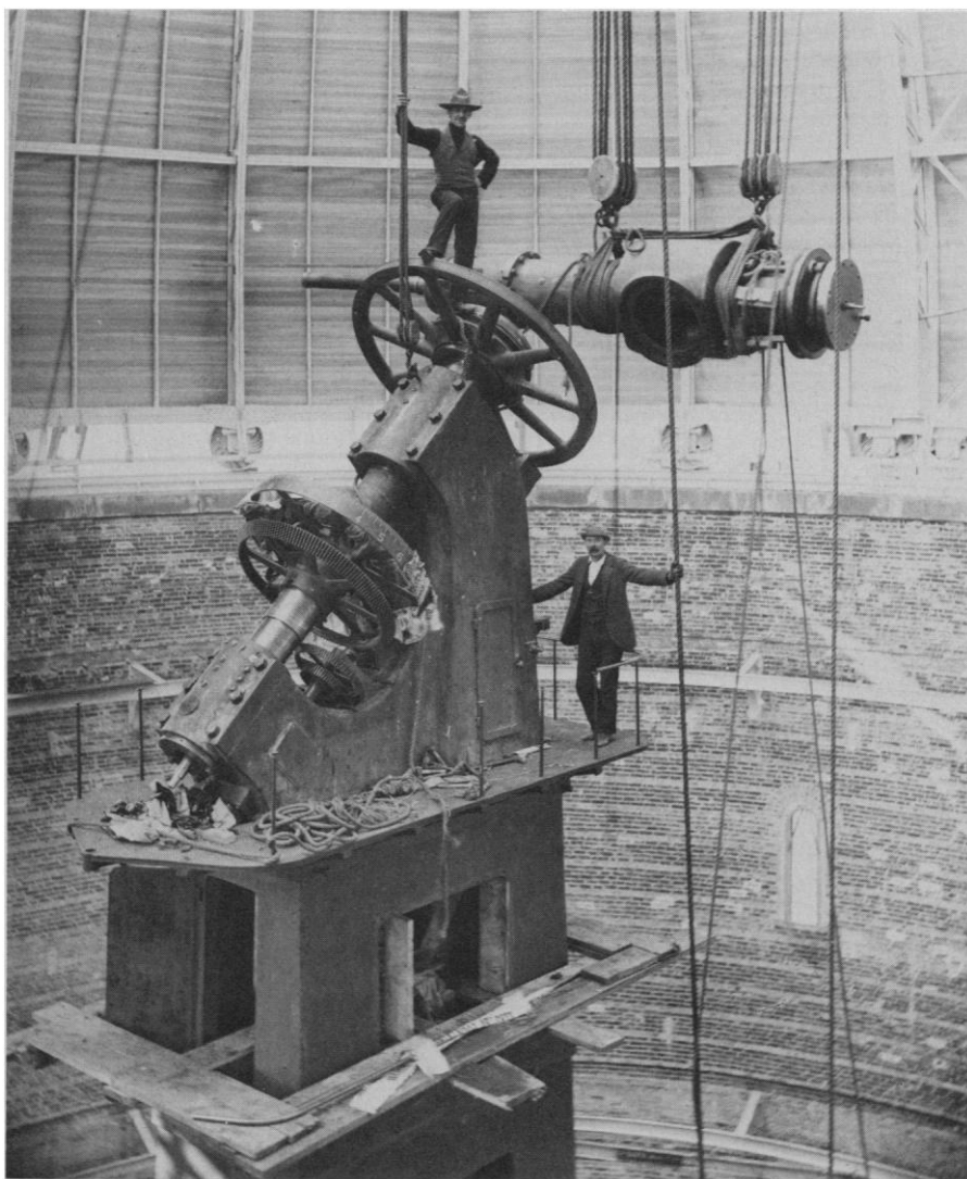
Installation of the mounting for the 40-inch telescope at Yerkes Observatory. [Yerkes Observatory photograph, University of Chicago, Williams Bay, Wisconsin; reproduced in Man Discovers the Galaxies ]
