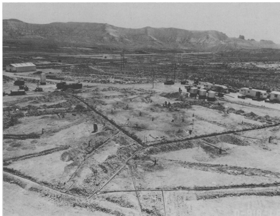
Fig. 3. The Laramie Energy Research Center's experimental in situ oil shale conversion site near Rock Springs, Wyoming. Each of the black pipes in the foreground is a well used for monitoring subterranean temperatures and water quality. [Source: U.S. Department of Energy]
